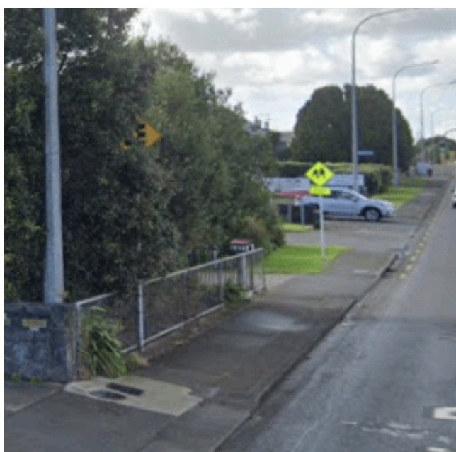
Figure 28: Showing road signs covered by vegetation.
